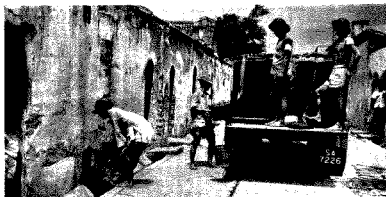
REMOVING THE SEWAGE.
